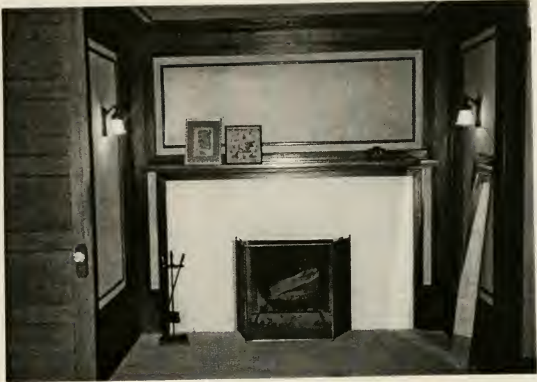
Figure 1.15 Restored Fireplace in master bedroom. Photograph by the author, 1999.
